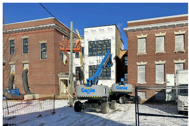
Construction on the connector between the two affordable housing apartment buildings
